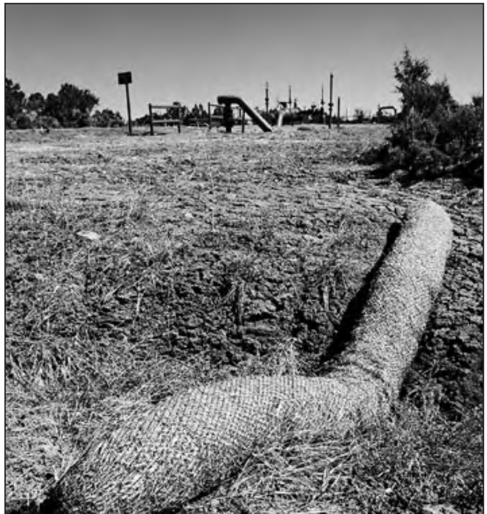
Simple erosion barriers, like this one below a natural gas well in on U.S. Forest Service land in the San Juan Basin, can help reduce the impact of energy development on habitat and wildlife by trapping sediment from stormwater runoff. (Joel Gay)
